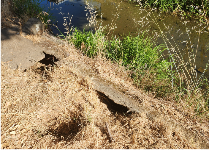
Figure 2: Site conditions at Tributary 2
