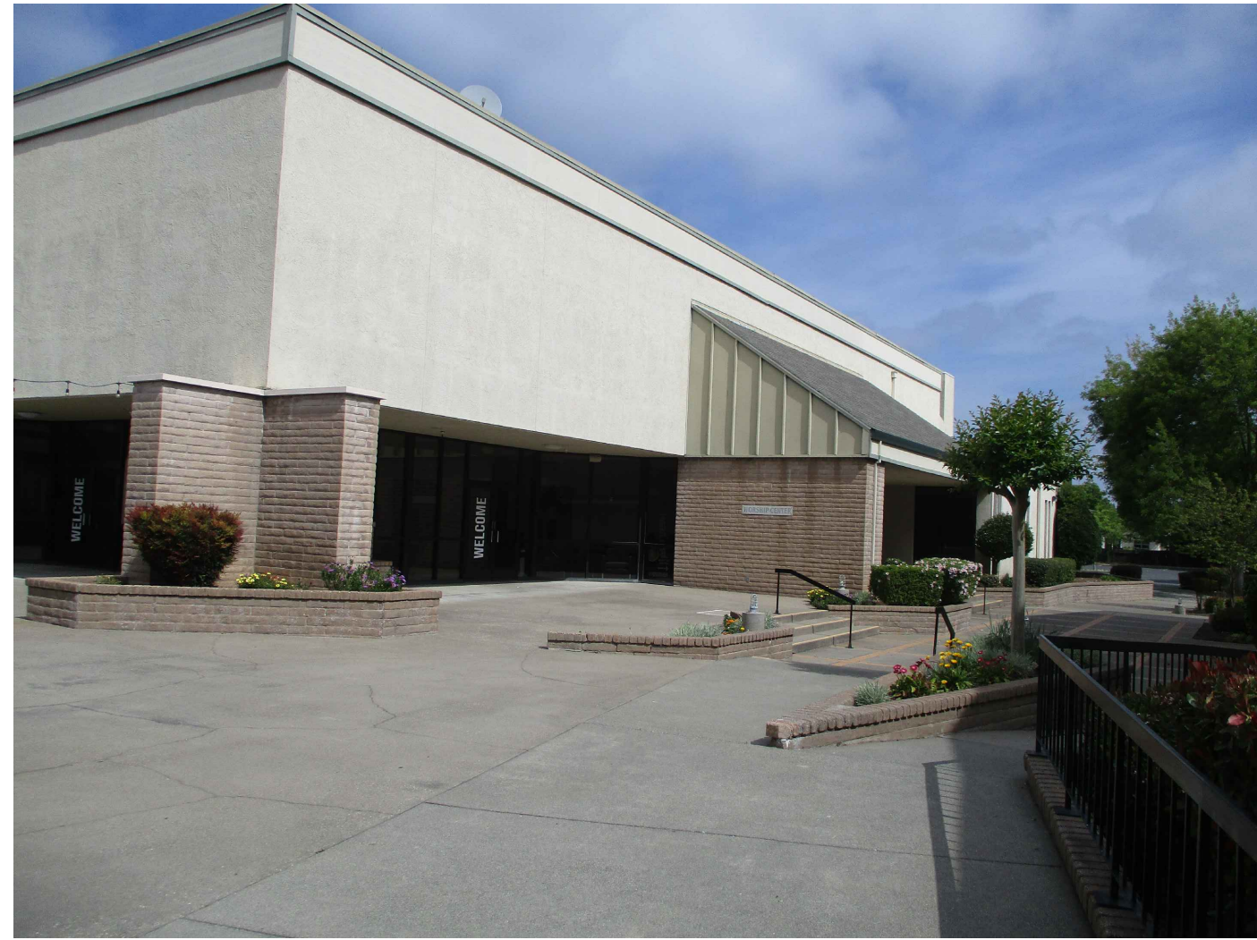
VIEW FROM COURTYARD
