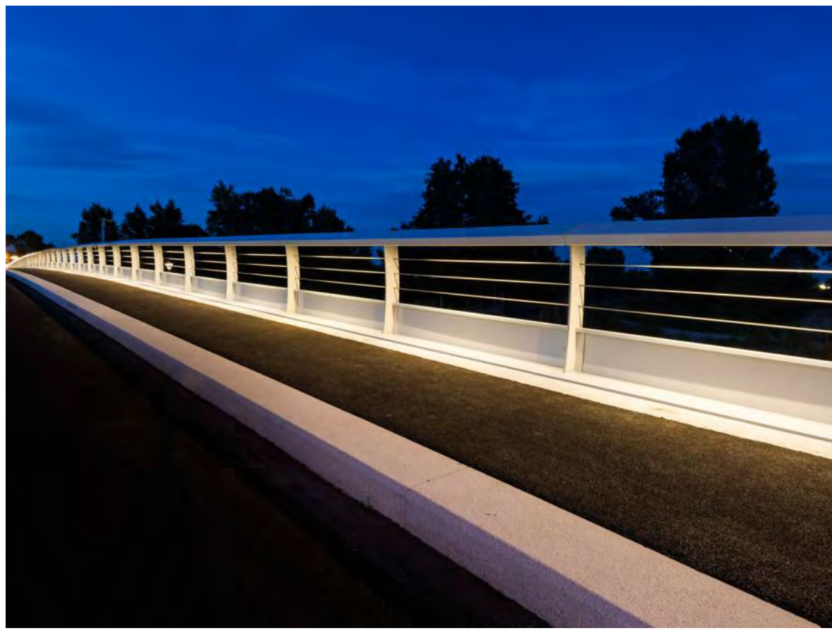
STRUCTURE AND OVERPASS LIGHTING
