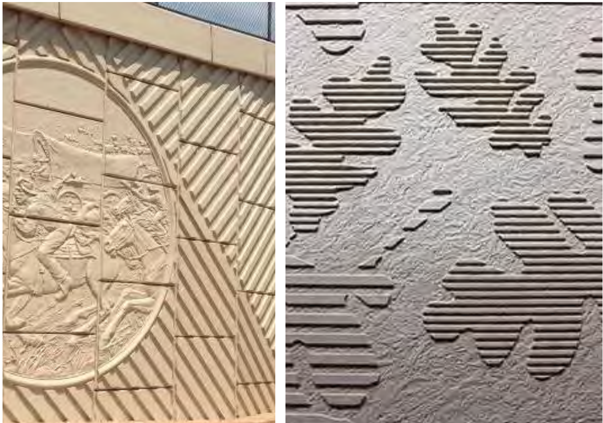
FORMLINER CONCRETE WALLS
