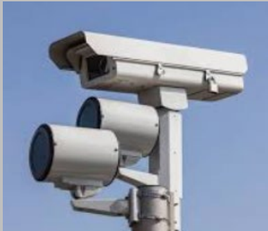
DOT Camera Upgrades (in-progress)
