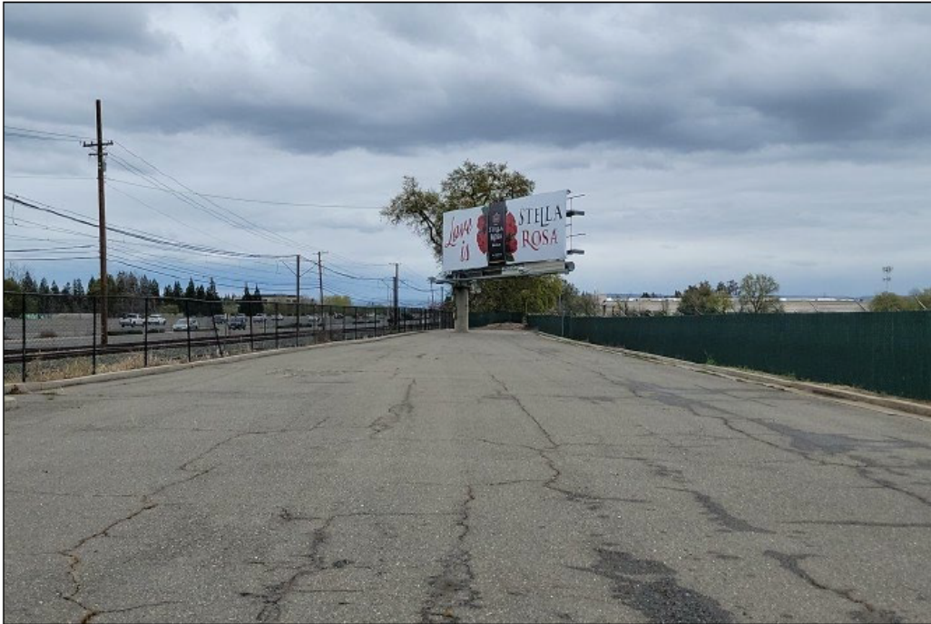
Figure 2: Existing Conditions (Looking East)
