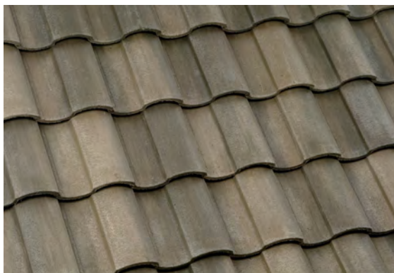
Roof: Eagle - 3687 Brown Gray Range
