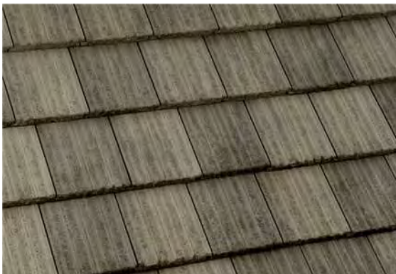
Roof: Eagle - 5687 Brown Gray Range
