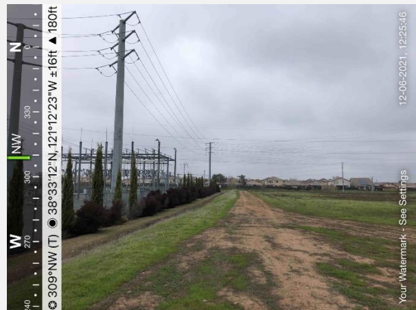
Photo 10. An unvegetated access road within the PSA and adjoining substation to the south.
