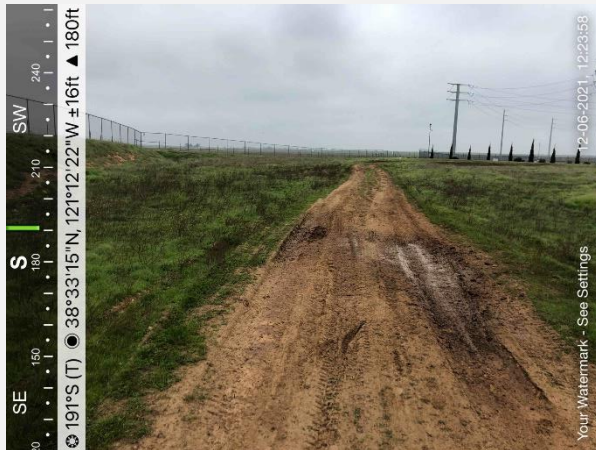
Photo 13. Road rut within PSA.
