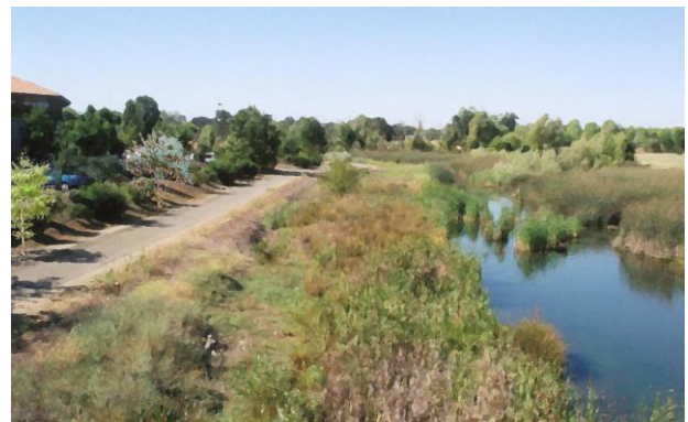
Example of naturalized drainage channel.
