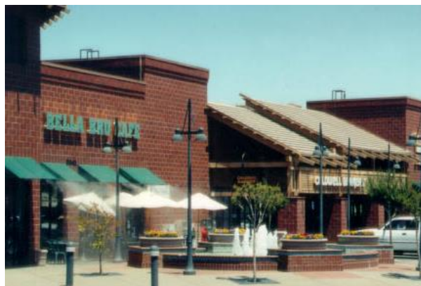
Cornice Detail and Variety of Roof Types
