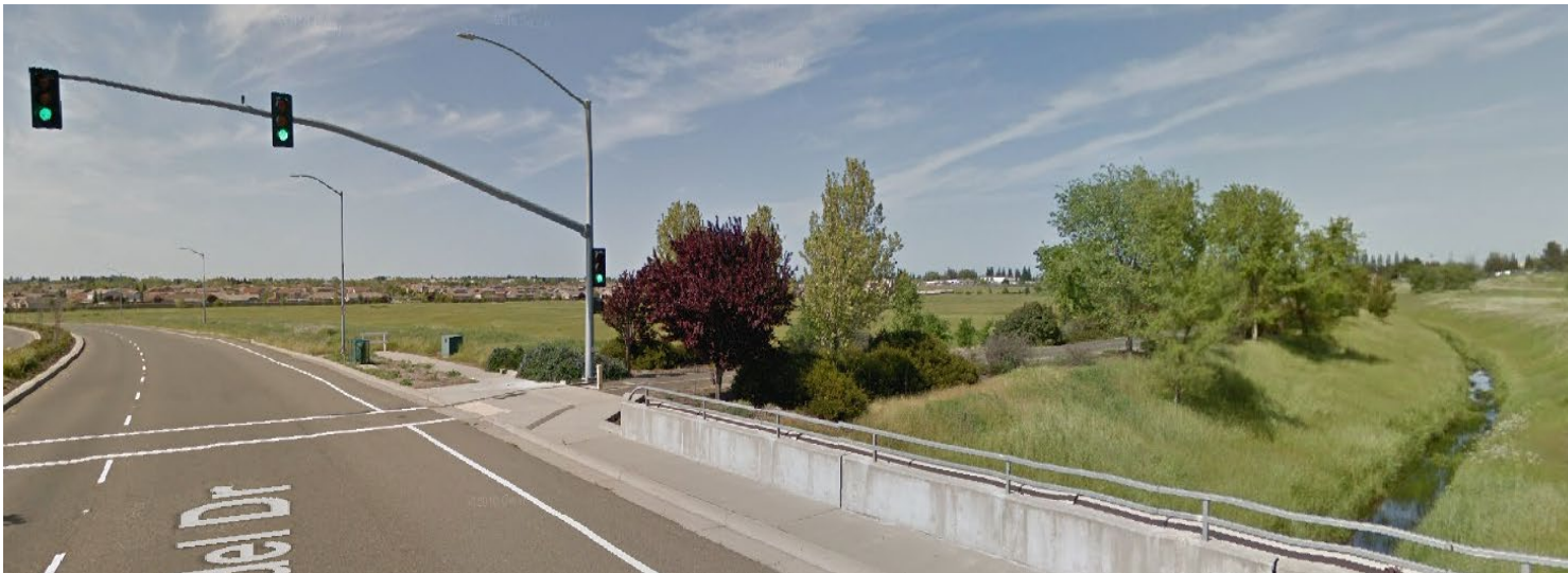
Zinfandel Drive Street View at the Pedestrian Crossing
