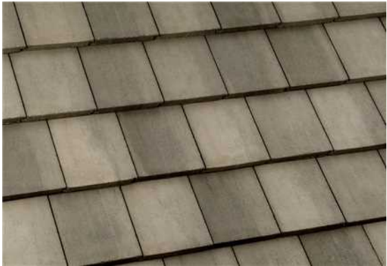
Roof: Eagle - 4687 Brown Gray Range
