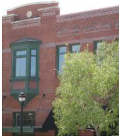
Flat Roof with Detailed Parapet
