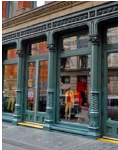
Storefront with Cast Iron Columns
