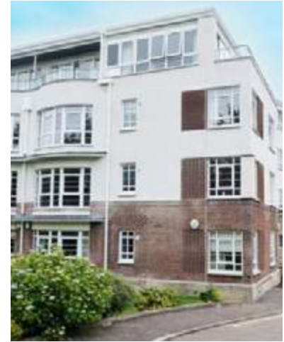
Scupper and Downspout on Side
