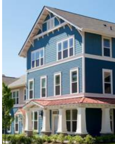
Bracketing a Roof Gable
