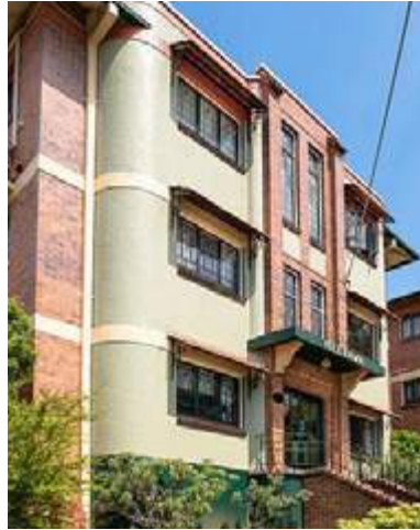
Gutter and Downspout
