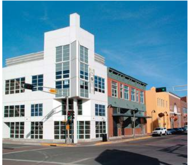
Liner Building with Garage Illustrative Photo
