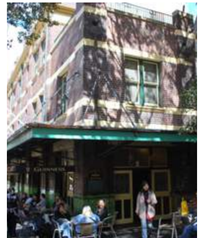
Commercial Frontage with Seating
