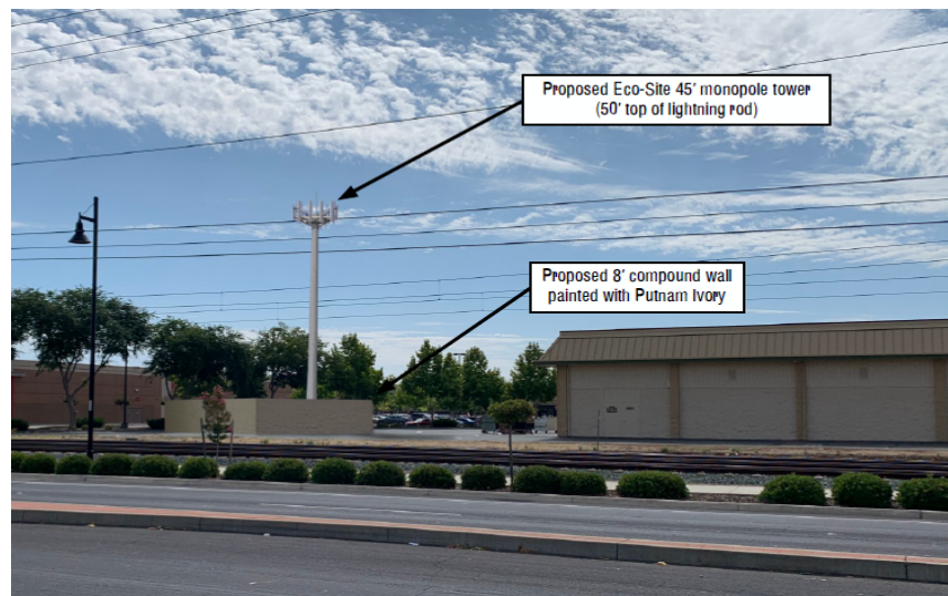
Figure 5: First Submittal Telecommunication Tower Designs
