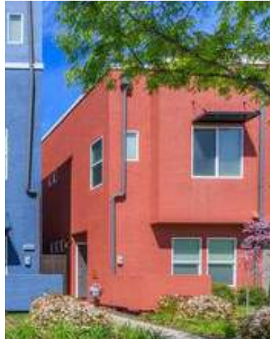
Scupper and Downspout
