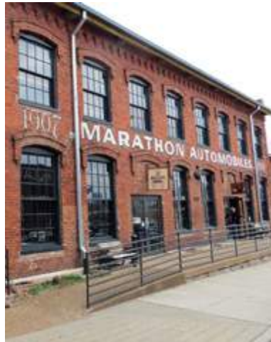
Two-Story Commercial Block
