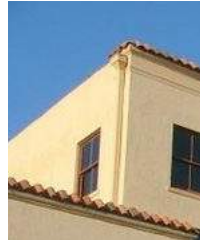
Scupper and Downspout
