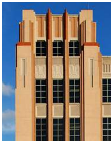
Column Extensions with Metal Panels
