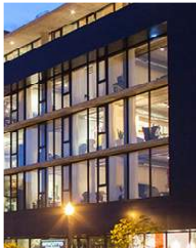
Windows Spanning Multiple Floors
