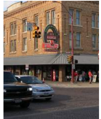
Awnings at Ground Floor Retail
