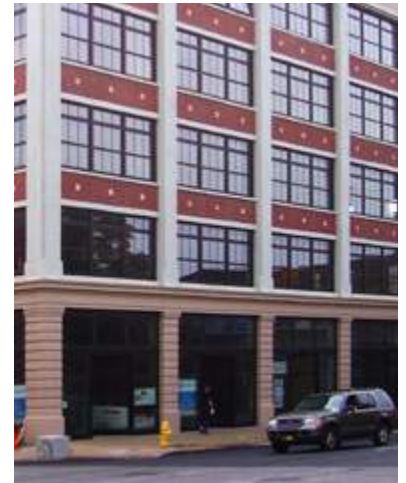
Large Windows Ground Floor
