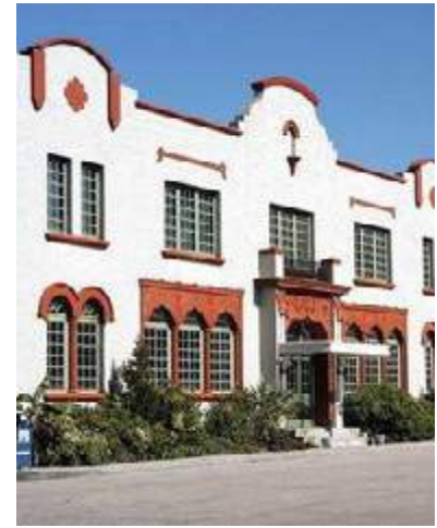
Parapet with Flat Roof
