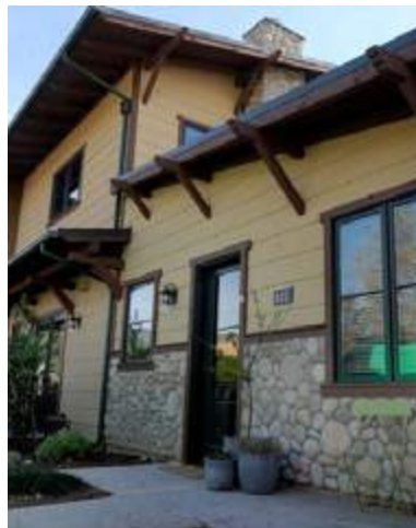
Brace and Exposed Rafters
