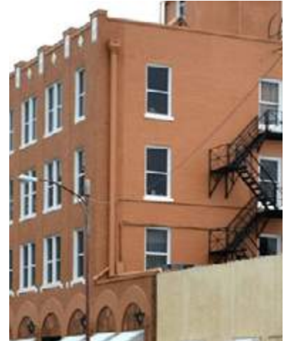
Drainage on Side of Building
