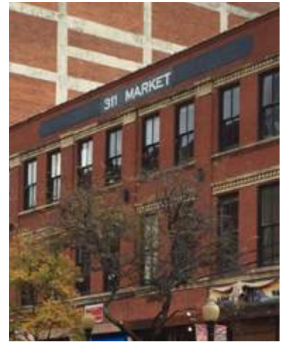
Parapet with Signage
