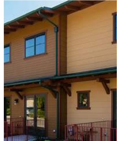
Gutter and Downspout
