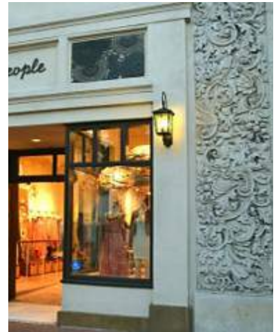
Appliqué at Cornice
