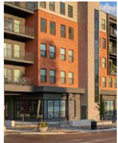
Openings Punched in Mass Wall
