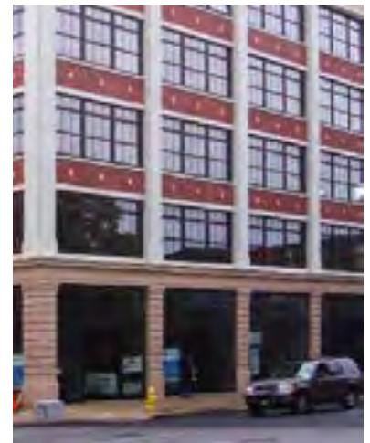
Large Windows Ground Floor
