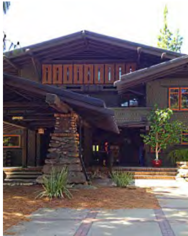
Upper Story Concealed in Roof
