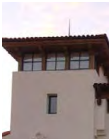
Expressed Rafters, Broad Eave
