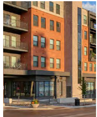
Openings Punched in Mass Wall
