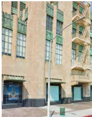
Masonry Base and Monolithic Wall
