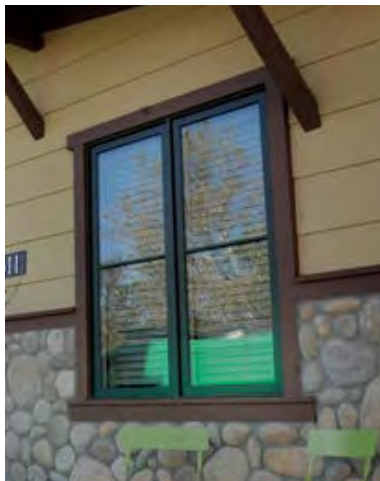
Paired Openings Composed Horizontally
