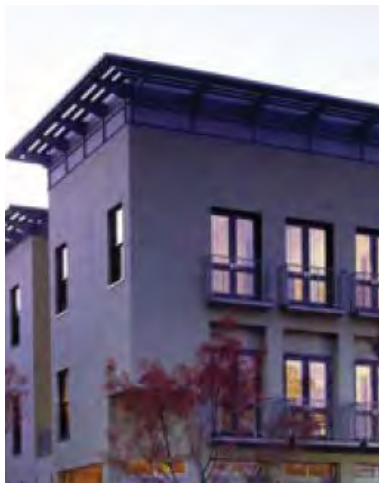
Roof Articulated with Raised Metal Overhangs
