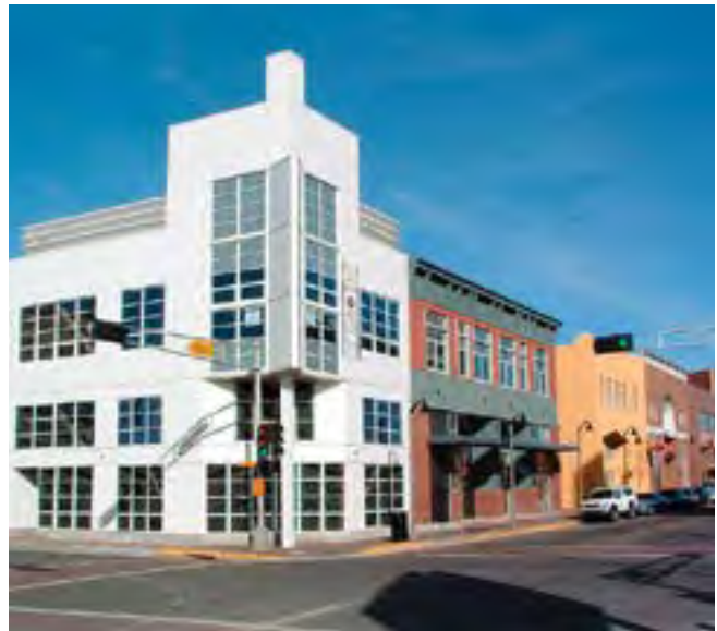
Liner Building with Garage Illustrative Photo
