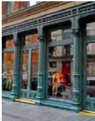
Storefront with Cast Iron Columns
