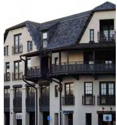
Dormer with Pitched Roof
