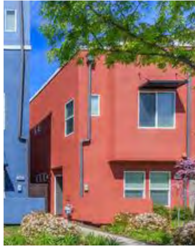
Scupper and Downspout
