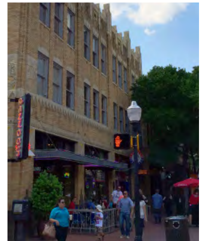
Awnings on Ground Floor
