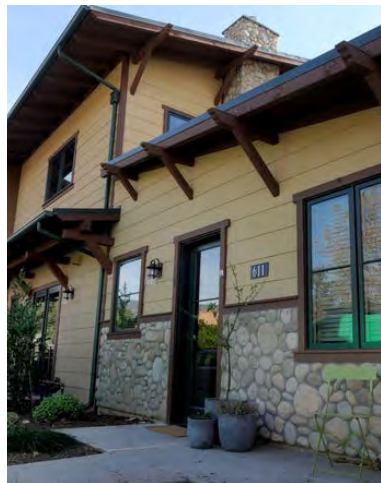
Brace and Exposed Rafters
