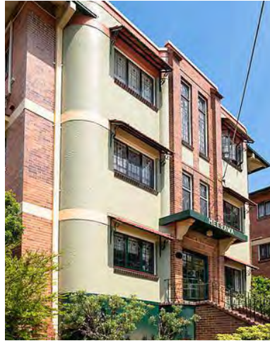
Gutter and Downspout
