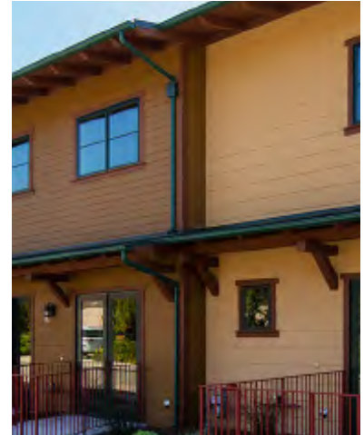
Gutter and Downspout
