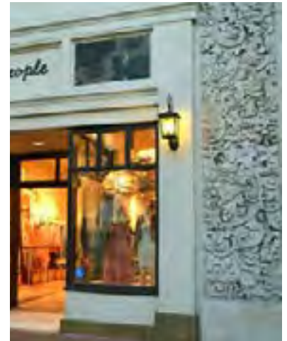
Appliqué at Cornice
