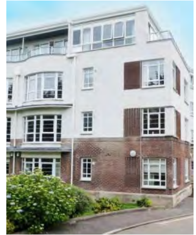
Scupper and Downspout on Side
