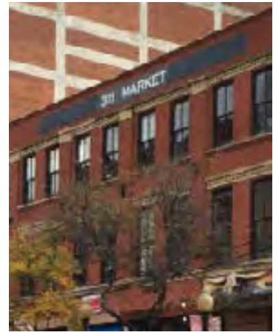
Parapet with Signage
