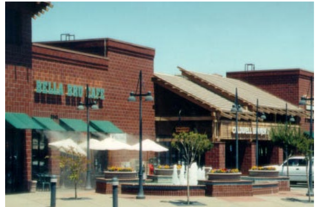
Cornice Detail and Variety of Roof Types
