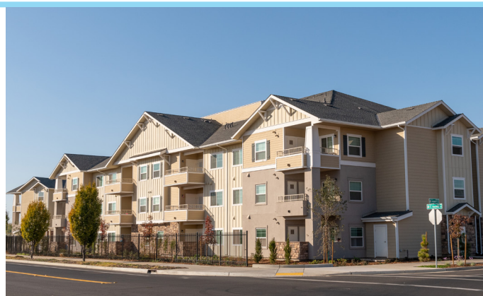
Bow Street Apartments – Elk Grove, CA.
