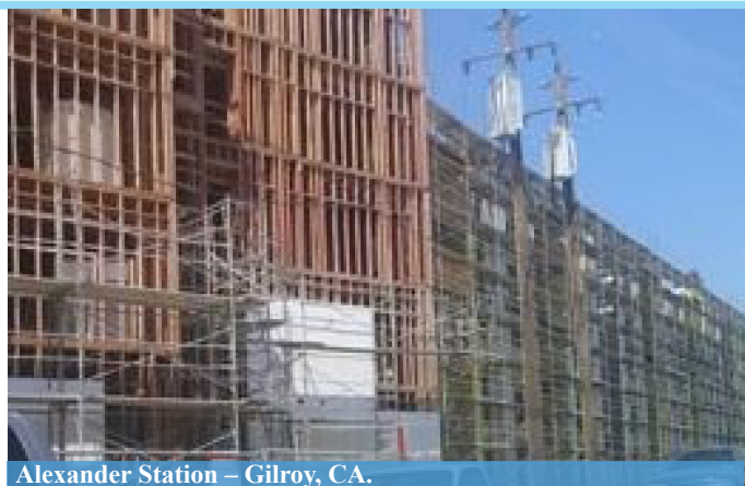
Alexander Station – Gilroy, CA.
