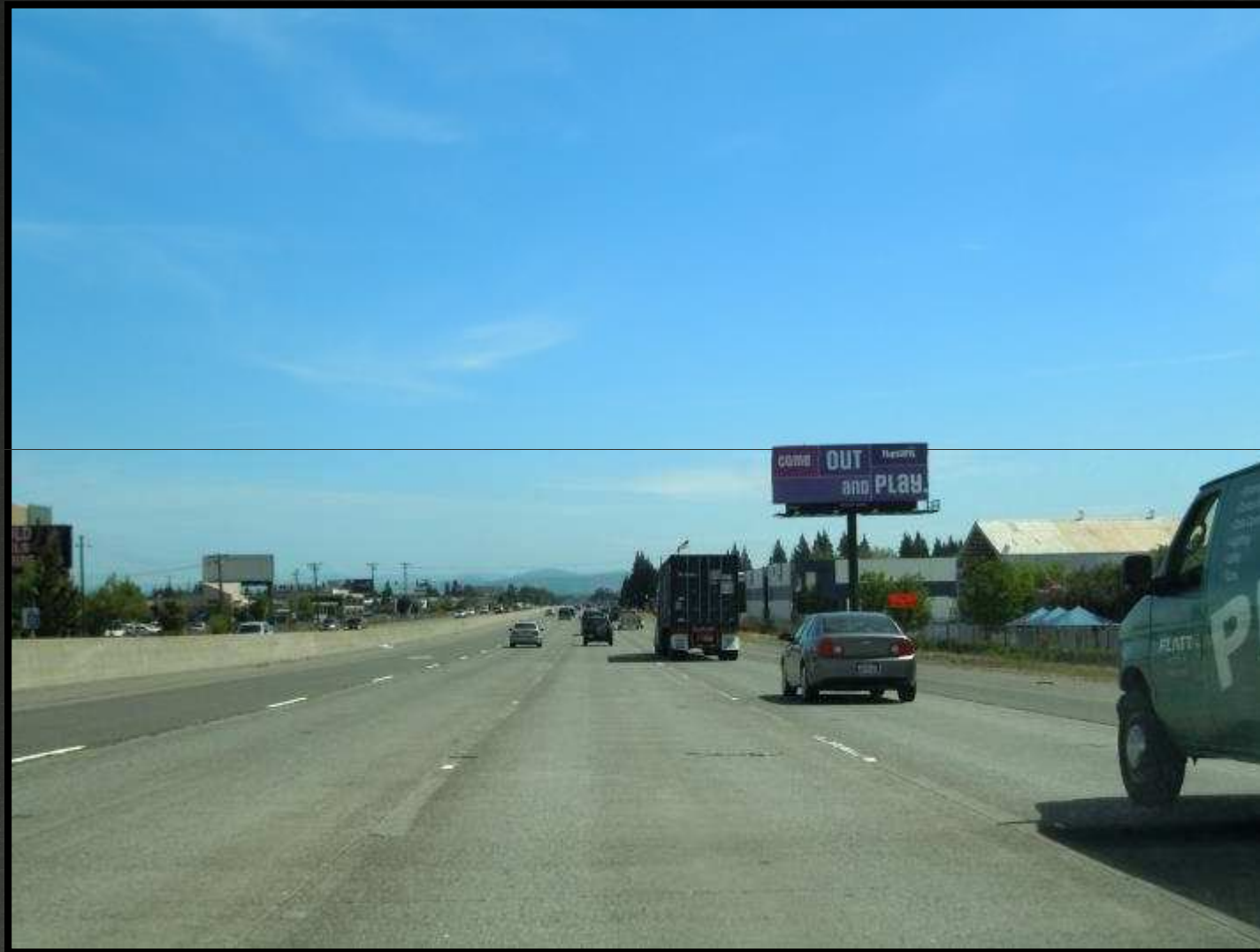
Rebuilt Sign – Highway 50
