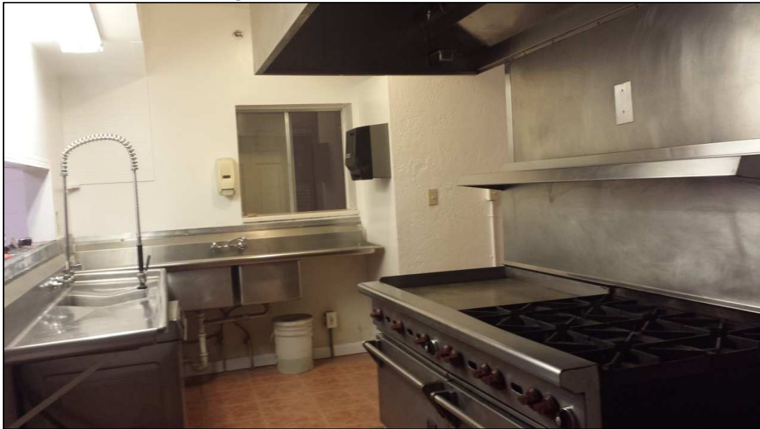
Figure 7 – Photo from Kitchen area
