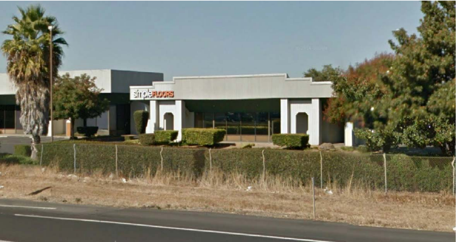
BUILDING B : AS VIEWED FROM THE SOUTH EAST
