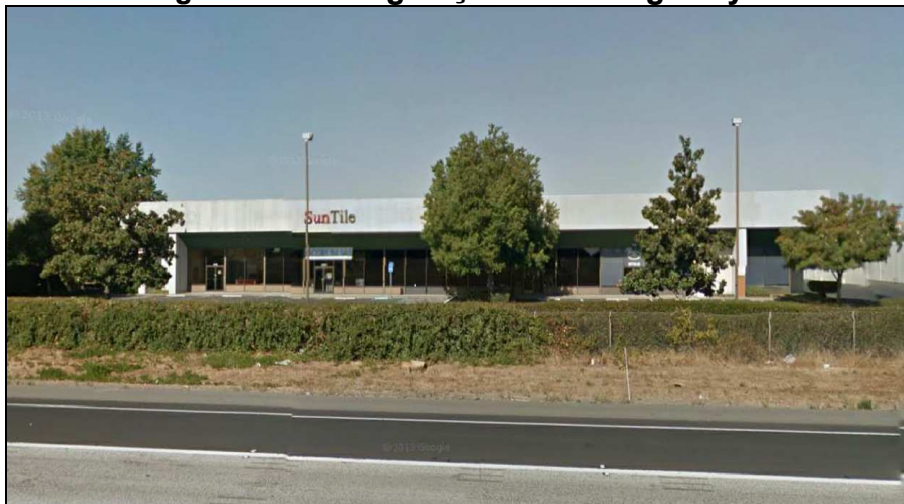
Figure 2: Existing Façade from Highway 50
