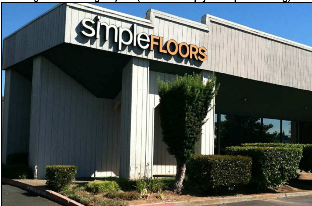
Figure 4: Existing Façade (faded T-111 plywood panel siding)
