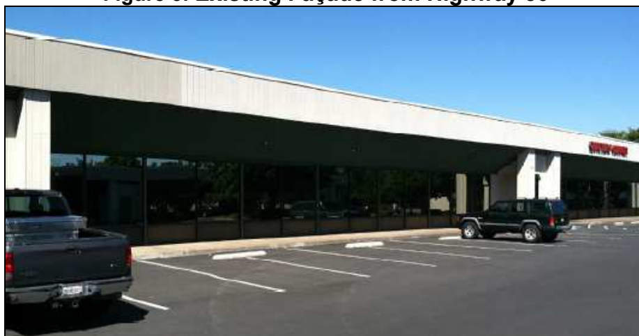
Figure 3: Existing Façade from Highway 50
