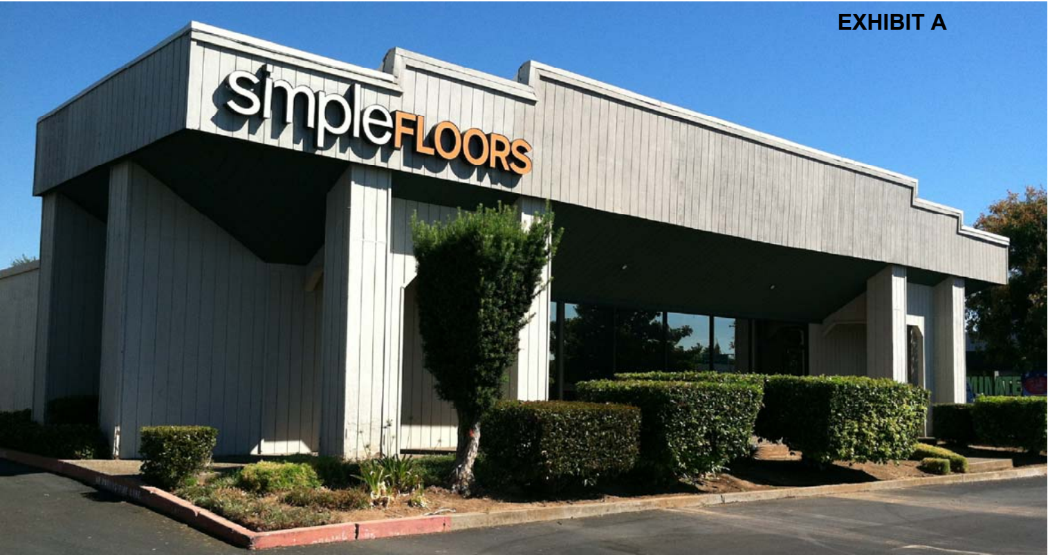
BUILDING B : AS SEEN FROM SOUTH WEST
