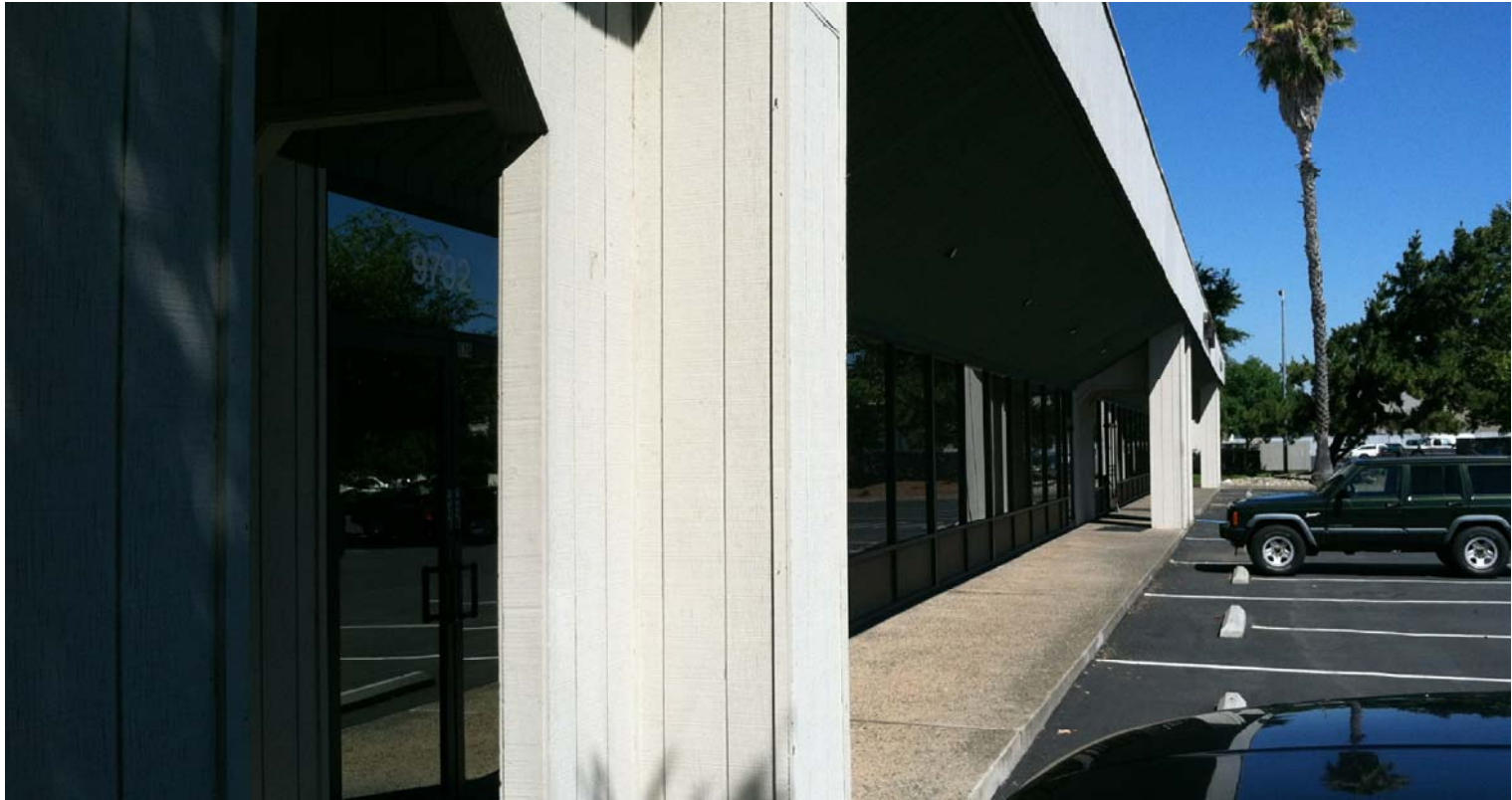
BUILDING B : DETAIL OF EXISTING T-111 SIDING
