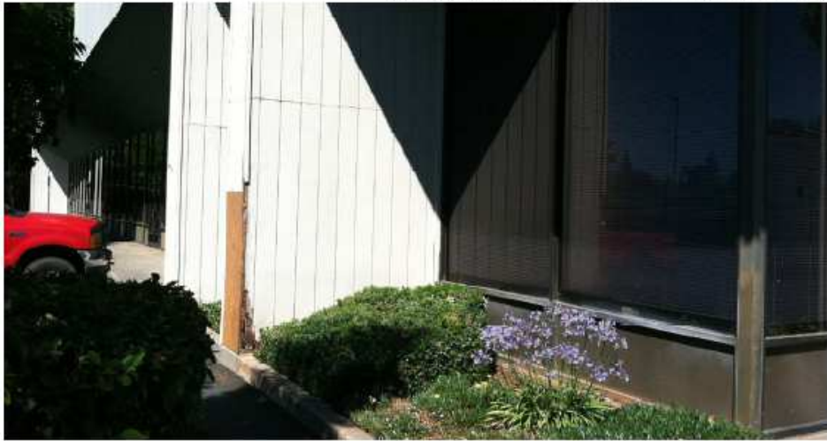
BUILDING A : DETAIL OF EXISTING T-111 SIDING
