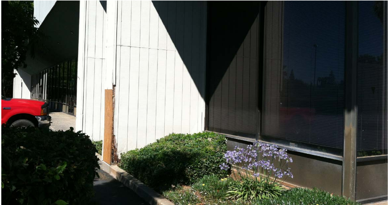
BUILDING A : DETAIL OF EXISTING T-111 SIDING
