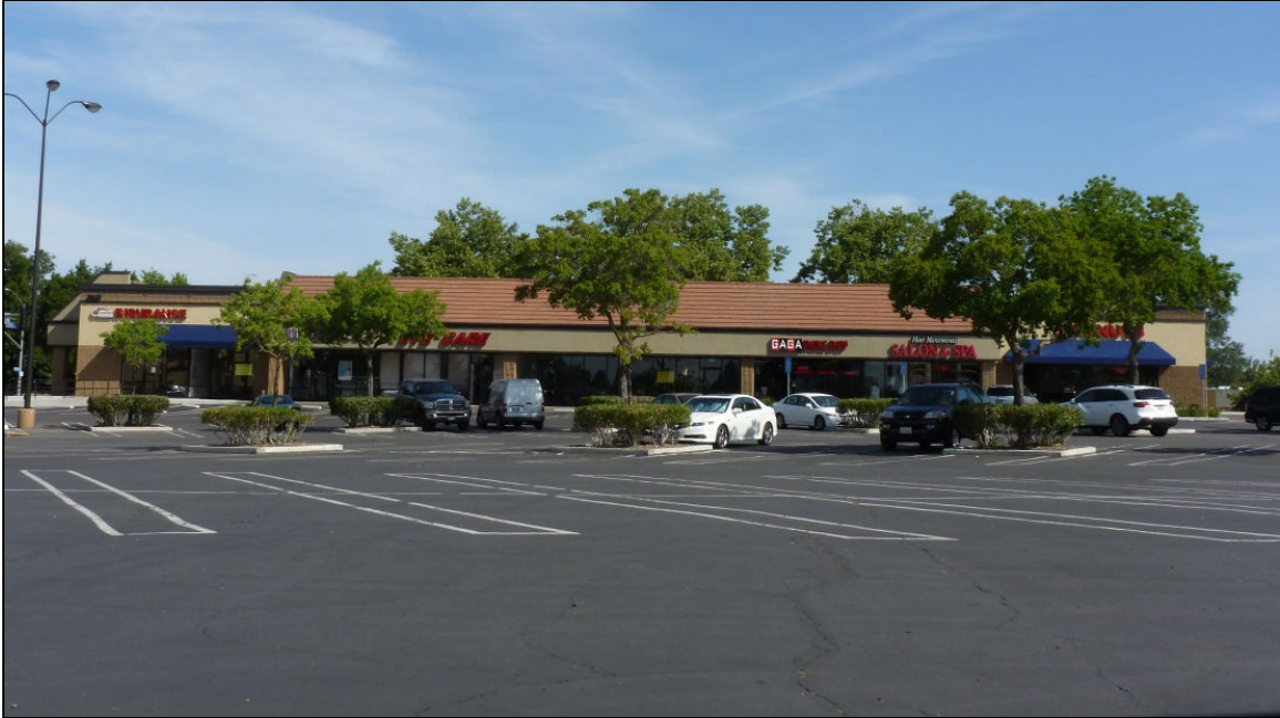
Figure 4: Photo looking at the existing commercial building on Parcel Four.
