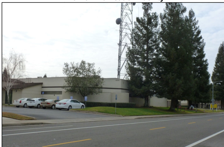
Figure 4: Photo from Systems Parkway looking West at the Sacramento County Fire Communication Facility
