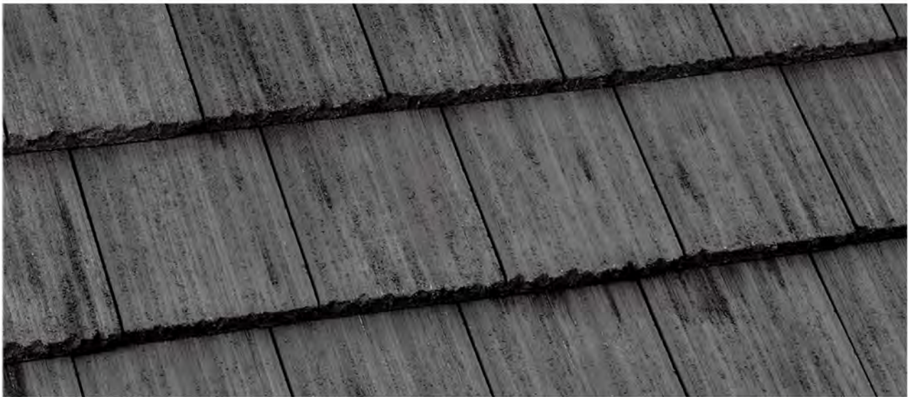
FLAT ROOF – EAGLE 5503
