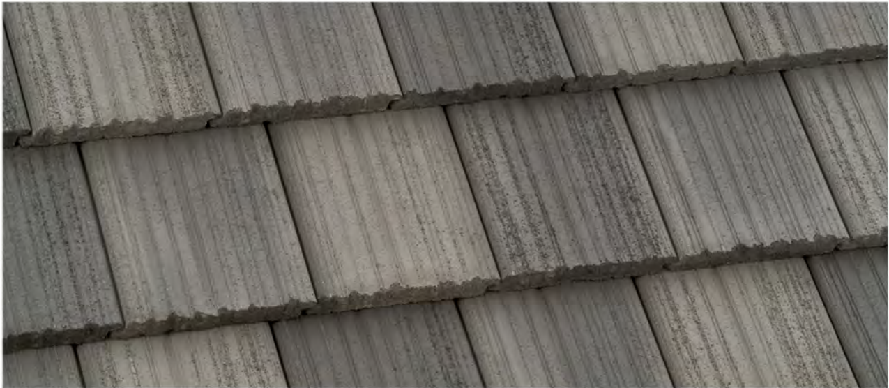
FLAT ROOF – EAGLE 5099
