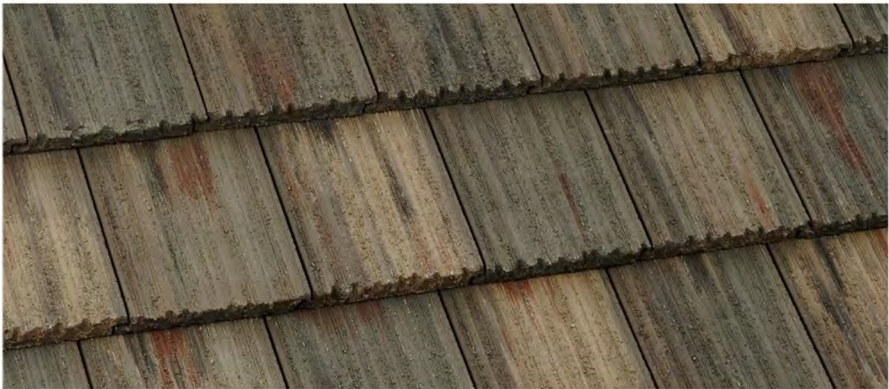
FLAT ROOF – EAGLE 5634
