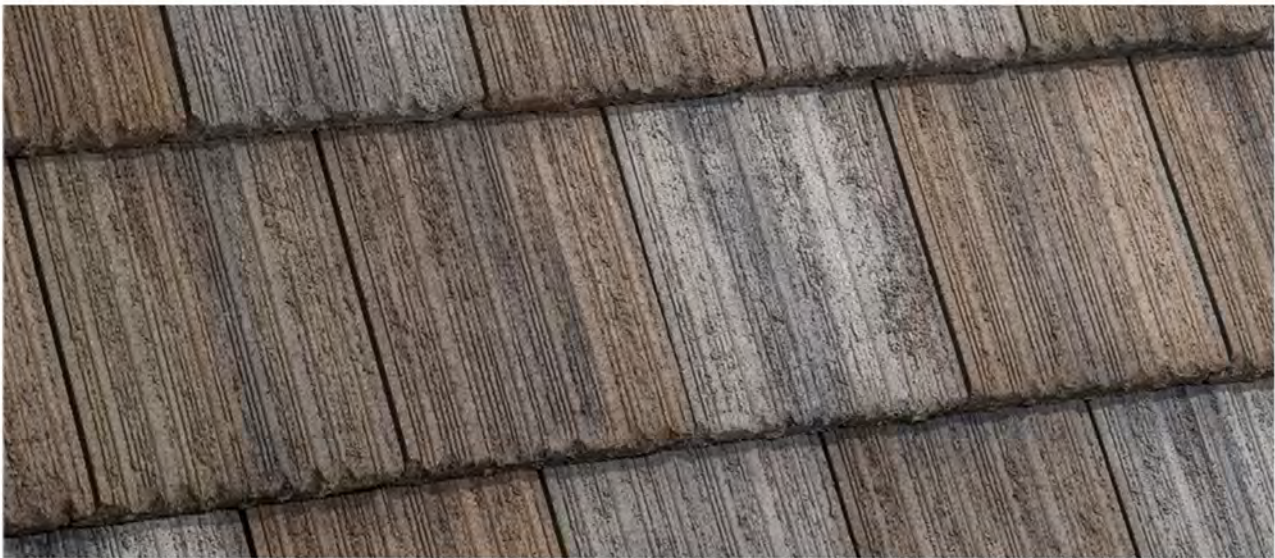
FLAT ROOF – EAGLE 5810
