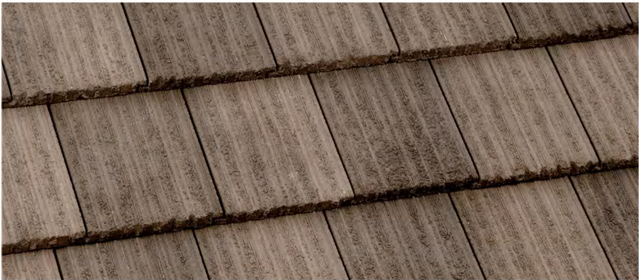
FLAT ROOF – EAGLE 5687
