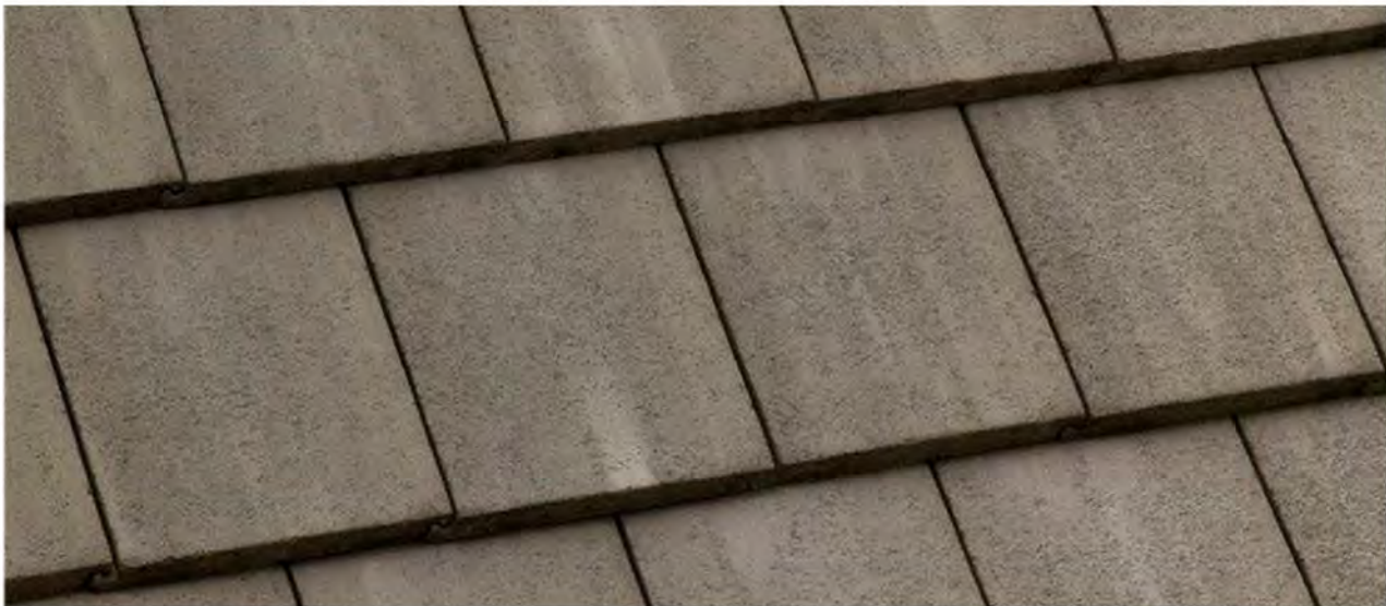
FLAT ROOF – EAGLE 4588
