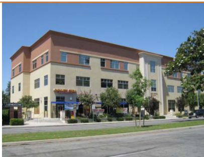
Offices over shops
