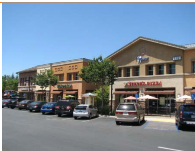
On-site main street
