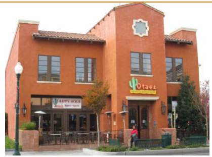
Offices over restaurant or retail
