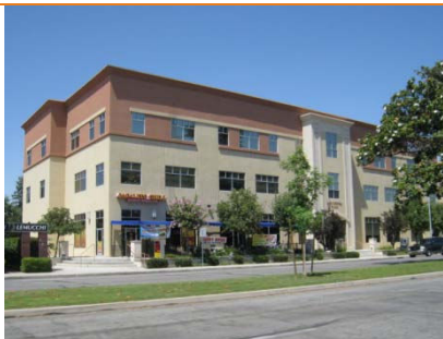
Offices over shops
