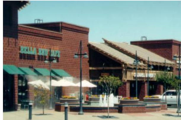
Cornice Detail and Variety of Roof Types
