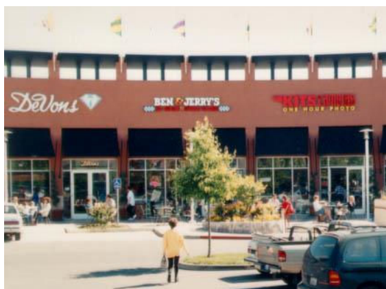
Windows, awnings, cornices and flags provide cadence.
