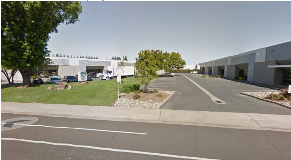
Figure 4: Photo looking north from Business Park Drive at the main entrance between the proposed Parcel Two and Parcel Three.
