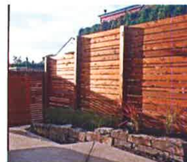
Because this fence had to step down a slope, labor costs were more expensive.
