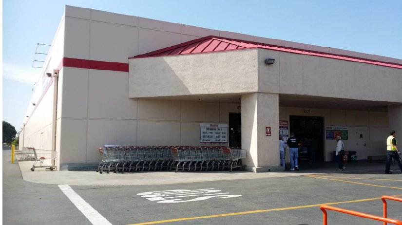
FIGURE 2: Existing Canopy at Entrance looking south
