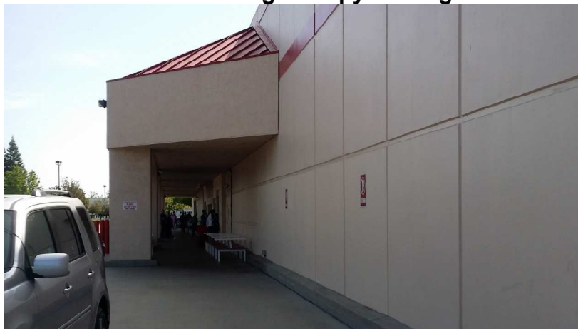
FIGURE 4: Existing Canopy looking east.
