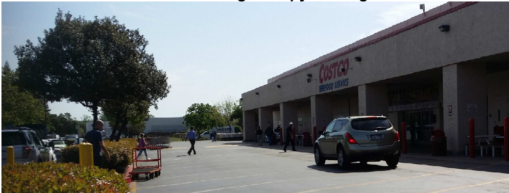
FIGURE 3: Existing Canopy looking east
