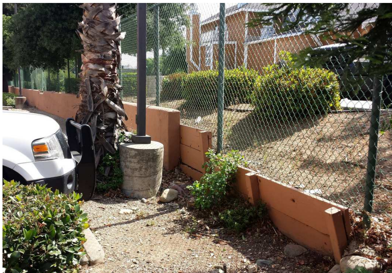
Figure 3: Existing Conditions (between existing Hyatt hotel and Fire Rock Grill)
