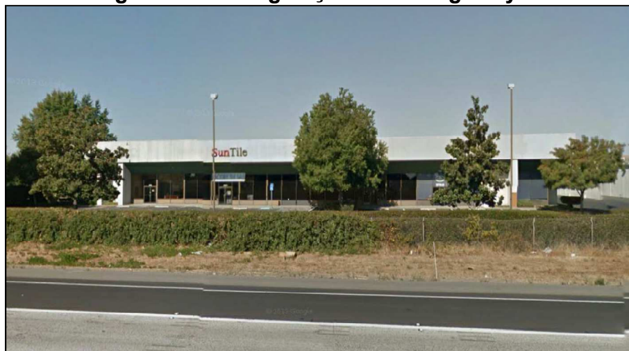
Figure 5: Existing Façade from Highway 50
