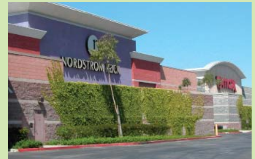
Rear of commercial buildings with screen wall
