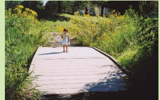
Bridge crossing over drainage channel
