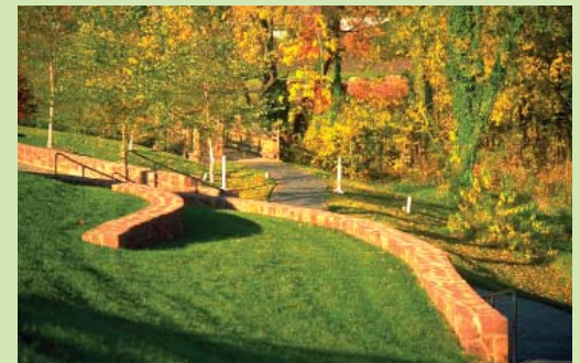
Decorative use of retention walls
