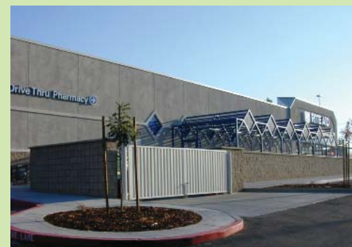
Service area hidden by architectural feature
