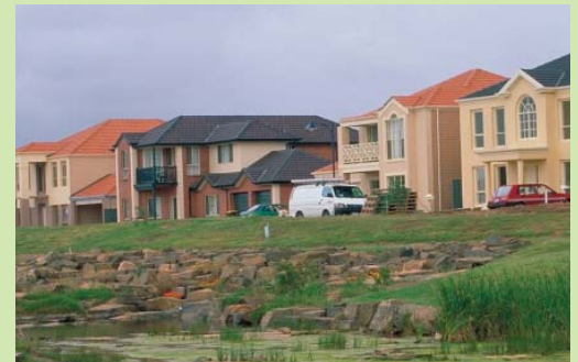
Natural drainage parkways
