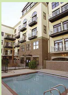
Courtyard view of podium unit © DESIGNLENS
