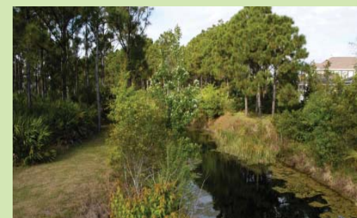
Naturalized drainage channel
