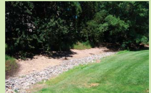
Drainage swale located at bottom of slope
