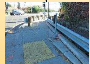
Chase/Coloma West Corner
