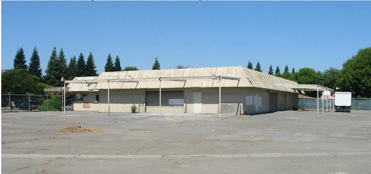
Figure 2: Previous building prior to Demolition
