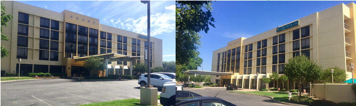
Figure 2: Main Entrance (South Elevation)
