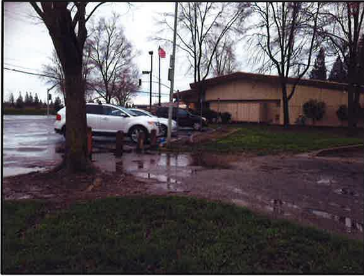
The project will address paving problems at the entrance to the Senior Center and Park.
