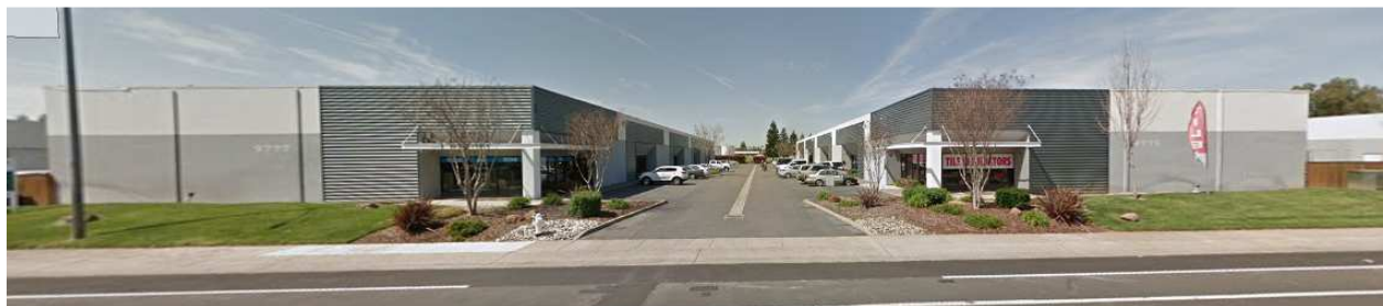
Figure 4: Existing Street View
