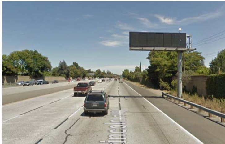
Figure 38 – Typical Freeway Changeable Message Sign (Xenon)
