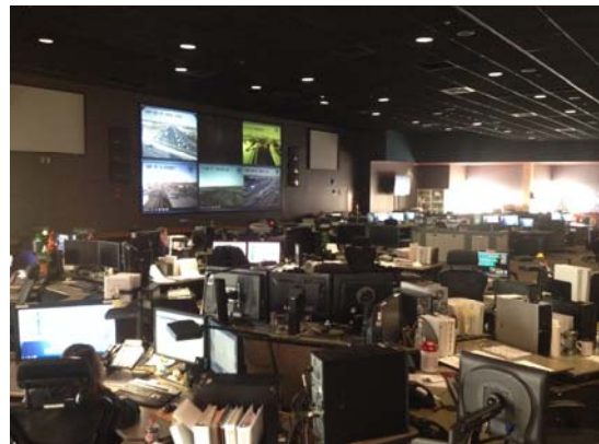
Figure 20 – Sacramento Regional Transportation Management Center
