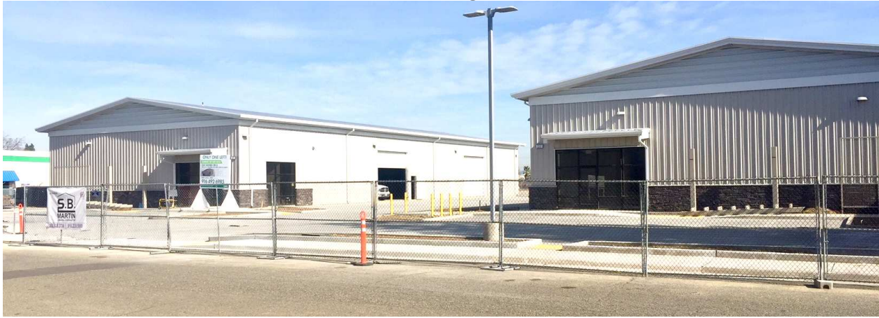
FIGURE 3: Existing Street View
