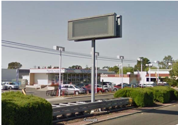
Figure 39 – Changeable Message Sign (2-sided) Operated by Sacramento County
