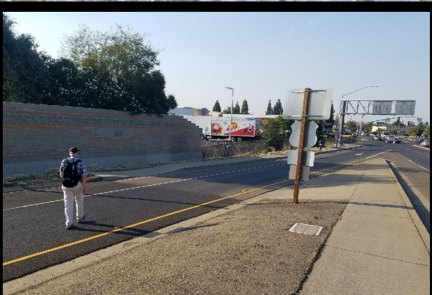
Lack of crosswalks at freeway ramps.
