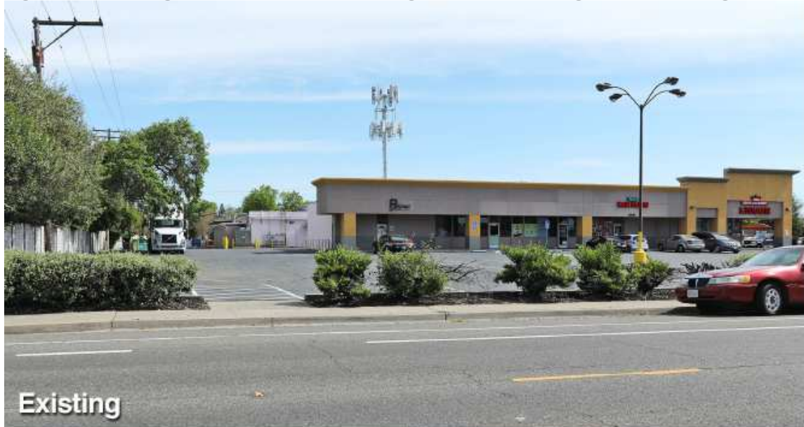
Figure 5: Existing Photo, Alternative Designs, and No Design from McGregor Drive
