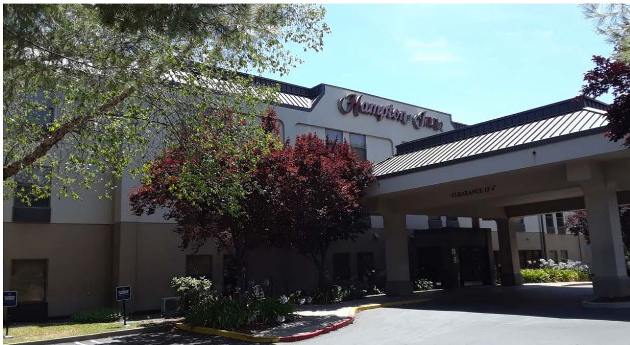
Figure 2: Existing Building Elevation (Main Entrance, Side and Rear Elevations)
