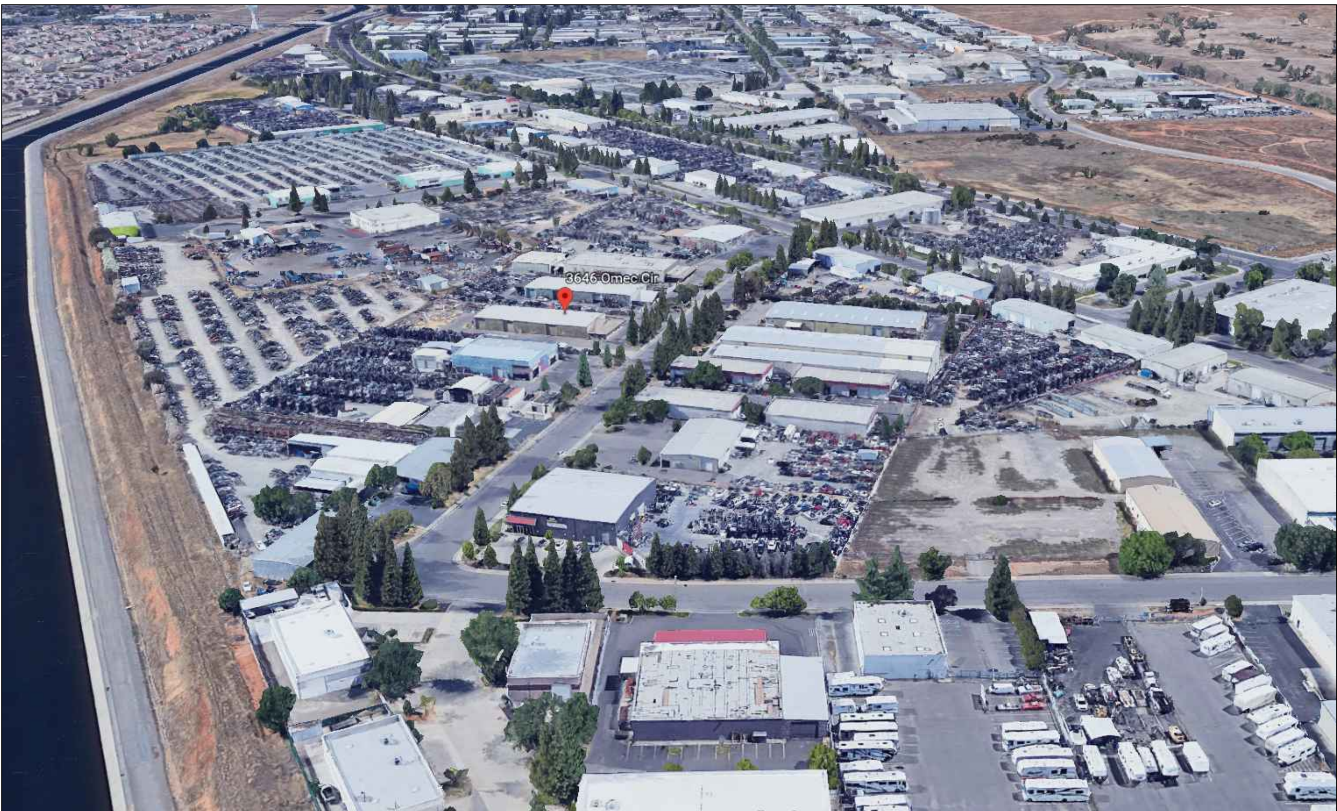
Aerial Vicinity 1 (Viewing North)
