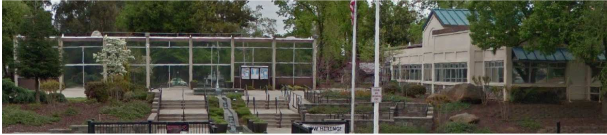
Figure 5: Existing Adjacent Buildings
