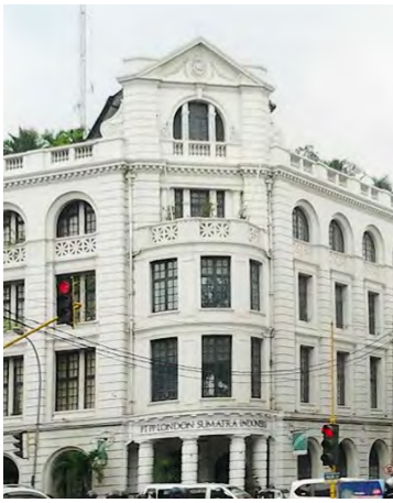
Balcony and Pediment
