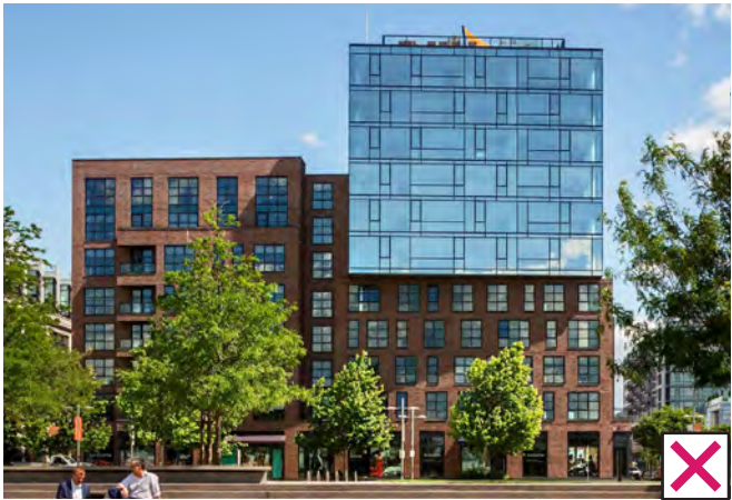
Facade Grid Incorrect / Inappropriate Glazed Mass Above
