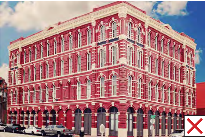
Excessive Amount of Facade Detail
