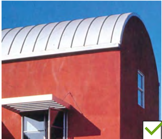
Metal barrel roof
