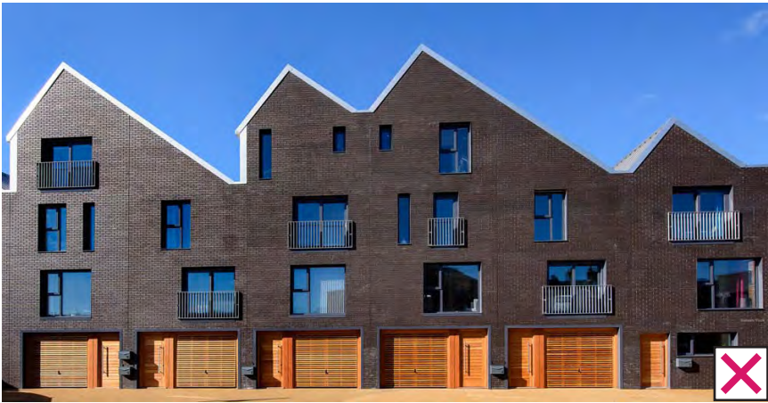
No Grid / Frame on Facade
