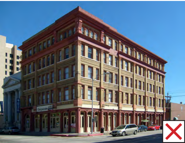
Excessive Amount of Facade Detail
