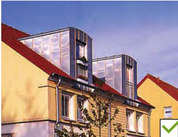
Sloped metal roof
