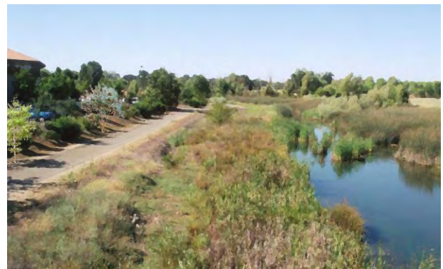
Example of naturalized drainage channel.
