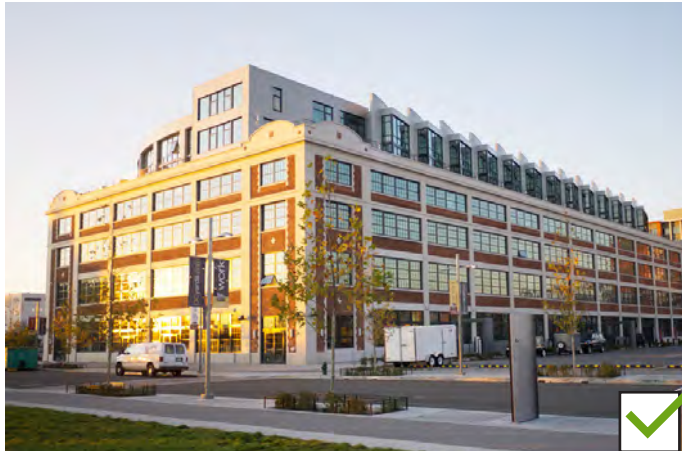
Utilitarian Massing Element on Top of Building Subordinate to Larger Composition Below
