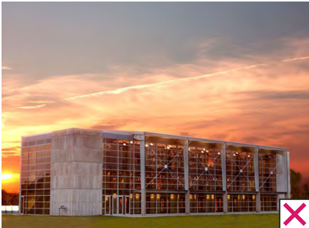
Too Much Glazing / Exposed Structure
