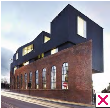
Abstract Mass on Top of Existing Structure Too Large
