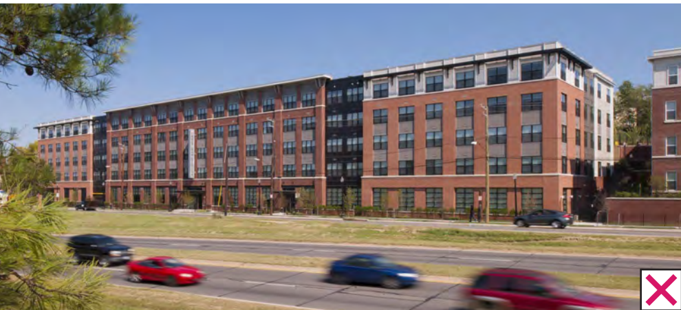
Inadequate Differentiation Between Facade Identities
