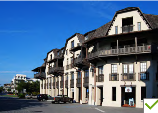
Appropriate Detailing / Organized Facade
