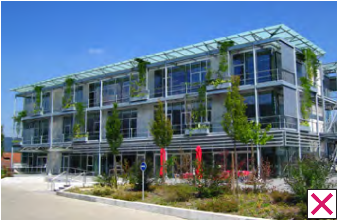
Unclear Vertical and Horizontal Grid on Facade
