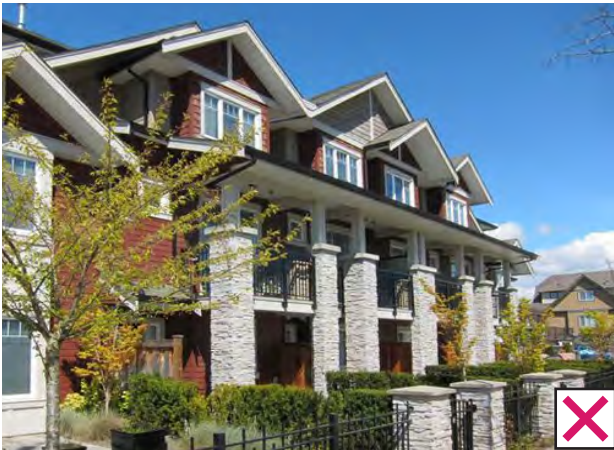
Too Many Roof Elements / No Brackets at Roof
