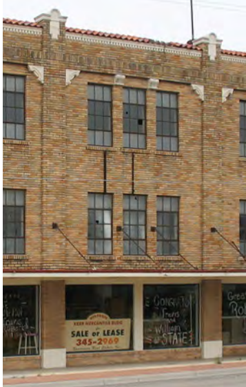
Awning over Large Openings at Ground Level
