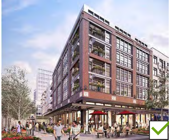
Clear Vertical and Horizontal Grid / Masonry Frame on Facade
