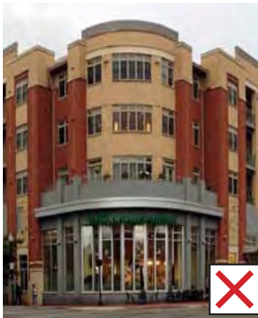
Inappropriate Material / Facade Plane Changes
