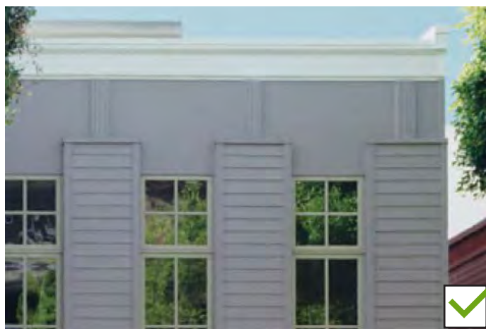
Parapet with cornice
