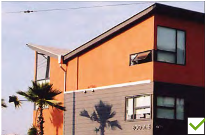
Plaster combined with siding
