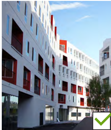
Clear Facade Composition with Simple Recessed Balcony
