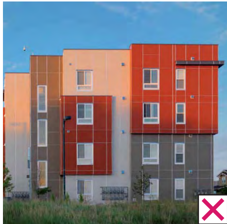
Disorganized Layering of Building Planes on Facade
