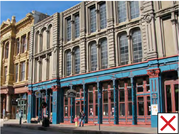
Scale of Space Above Ground Level Too Large
