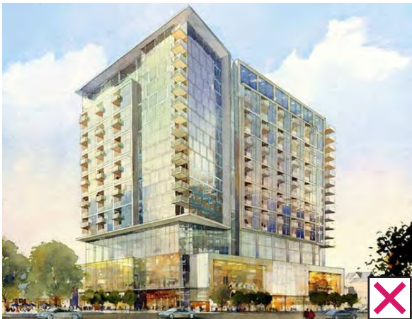
Overly Excessive Glazing / Expensive Structural System
