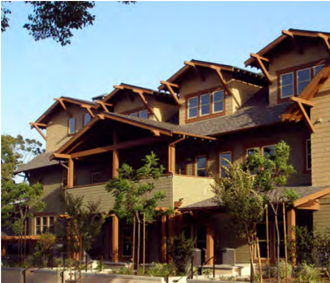
Examples of Brackets on Roof Dormers / Extended Balcony off of Facade
