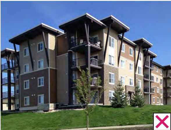
Building Detail out of Scale / Awkward Detailing
