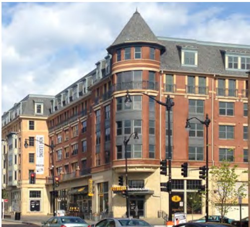
Pronounced Turret at Corner
