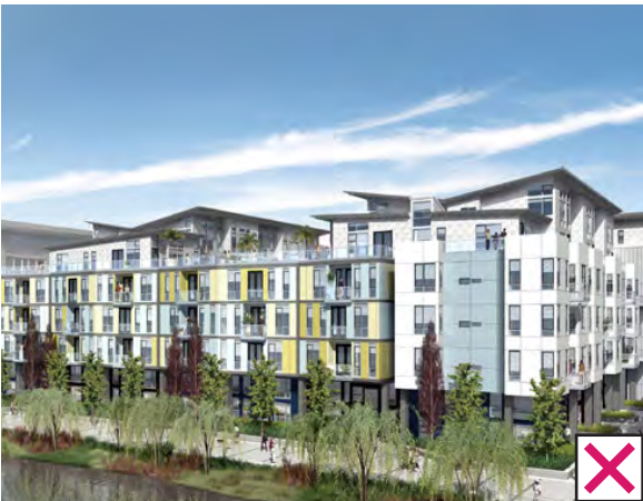
Elaborate Detailing / Fenestration, Structural system
