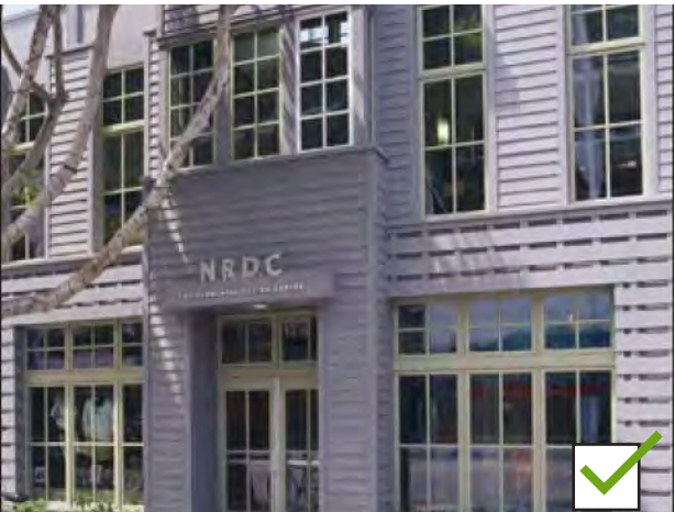
Painted Hardiplank siding
