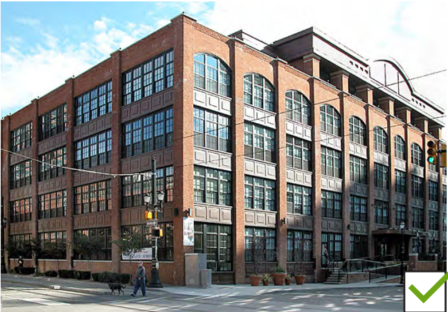
Simple Structural Grid / Frame On Facade
