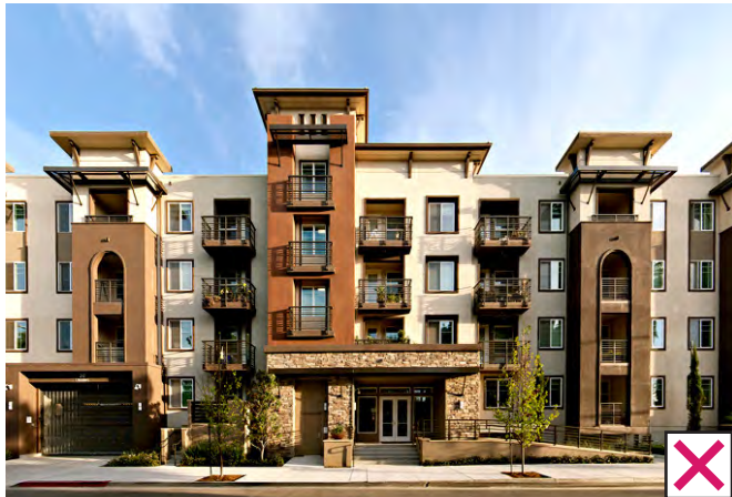
Incorrect Detailing / Strange Massing Moves
