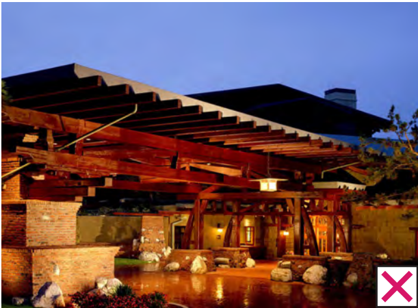
Excessive Bracket Detailing / Awning Too Large
