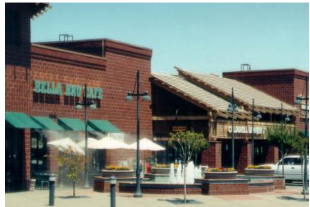
Cornice Detail and Variety of Roof Types
