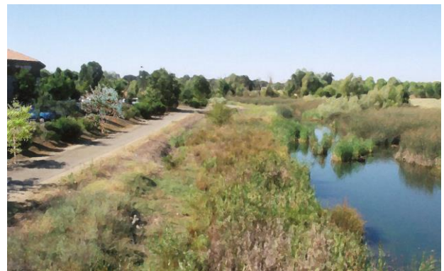
Example of naturalized drainage channel.
