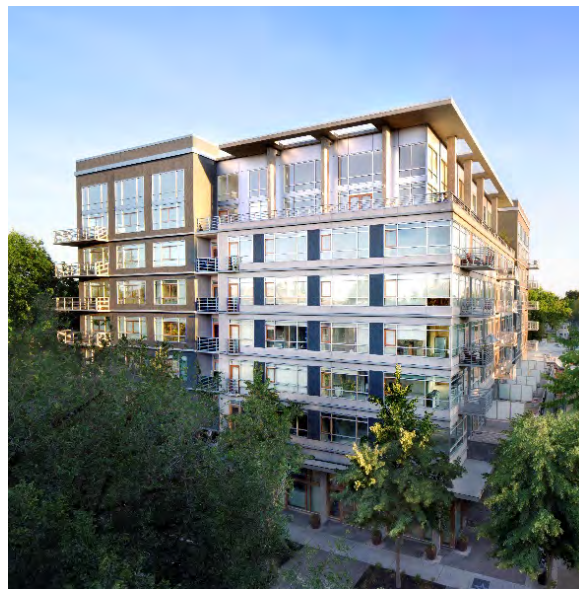
L STREET LOFTS
