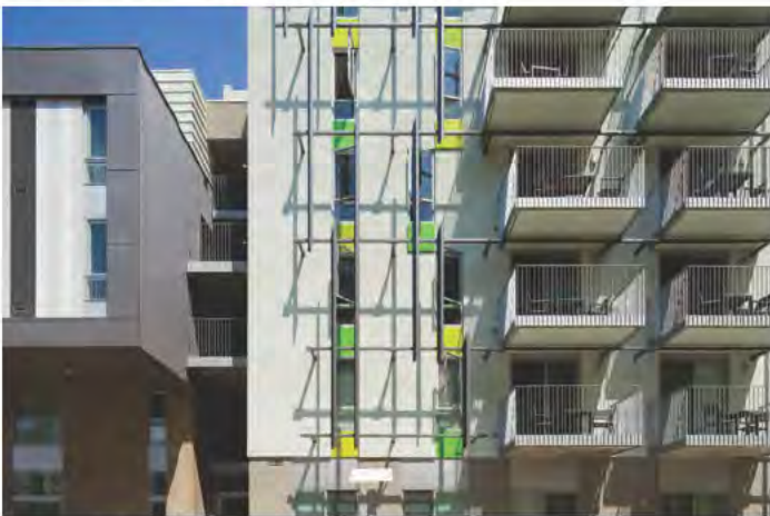
Community Great Room Facade
