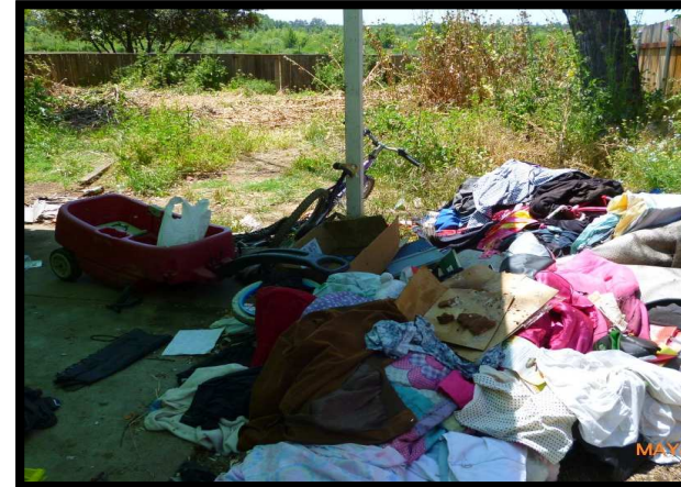
Electrical tampering & accumulation of garbage
