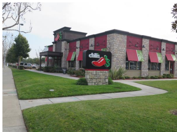
Buildings face the street along major arterials
