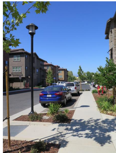
Minor Residential Street with landscaped bulbouts and pedestrian-scale lighting
