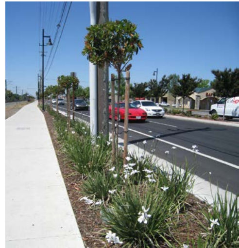
Continuously landscaped area between sidewalk and street along nonresidential collector streets
