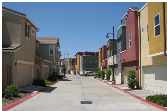
Alley provides rear access
