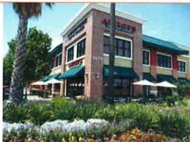
Offices over shops and restaurants
