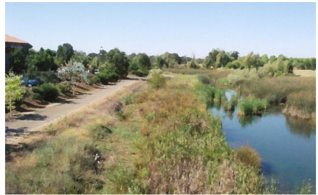
Example of naturalized drainage channel.
