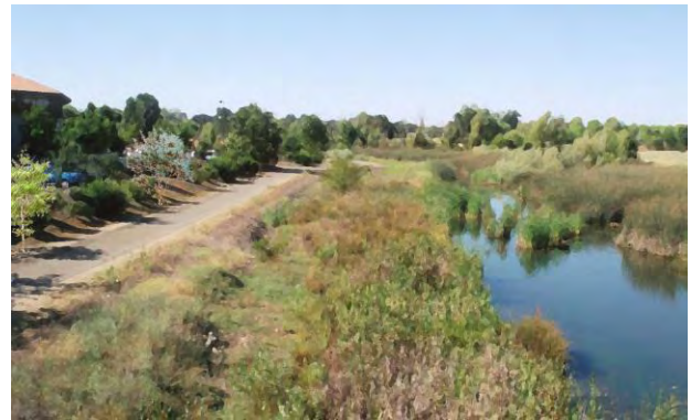
Example of naturalized drainage channel.
