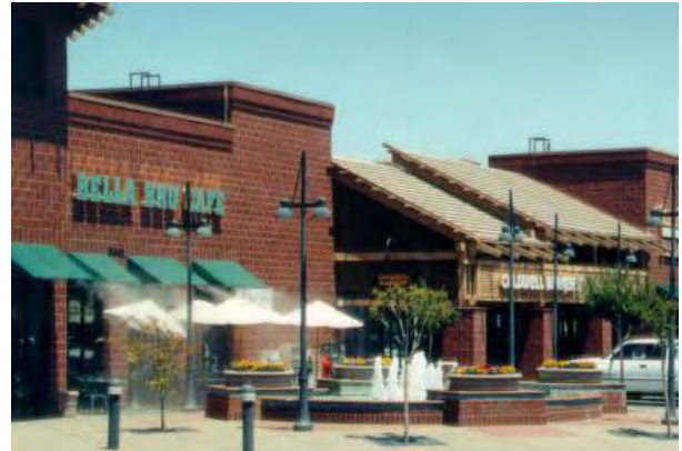
Cornice Detail and Variety of Roof Types
