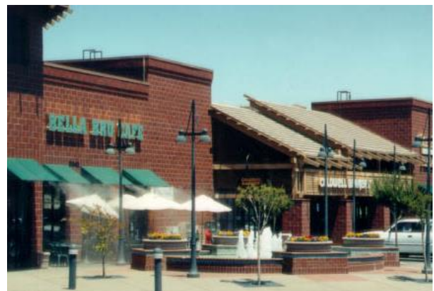
Cornice Detail and Variety of Roof Types
