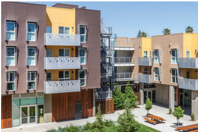
Exterior elevation with courtyard
