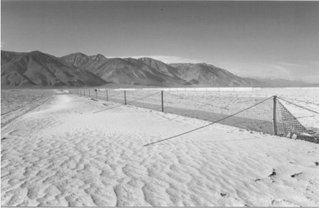
3002 3003 Figure 14-2. Sand fences (seven sets visible) early in the SLC UC Davis mitigation 3004 project.
