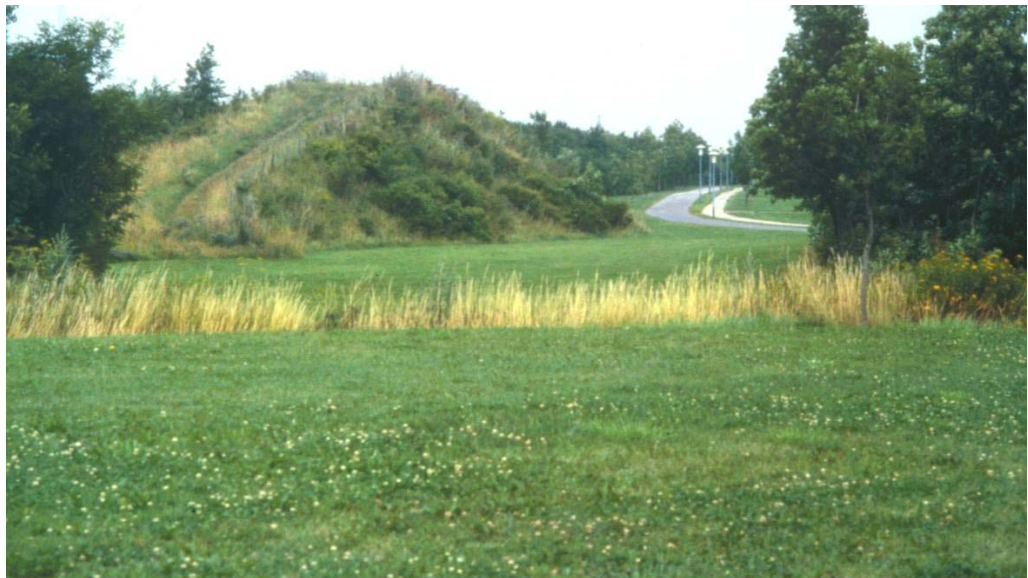
Figure 6.7. Earth embankment with a path on the top designed to fit into the urban landscape along a highway. Earth embankments can be made of surplus soil from road or housing construction projects in the region where a plan for the earth embankment is made and over a period of many years, dirt is delivered to the site before the embankment is finished. It is important to have a plan for the embankment in order to get a good final appearance in the visual environment.
