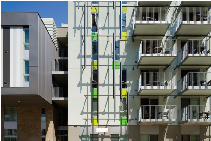
Community Great Room Facade
