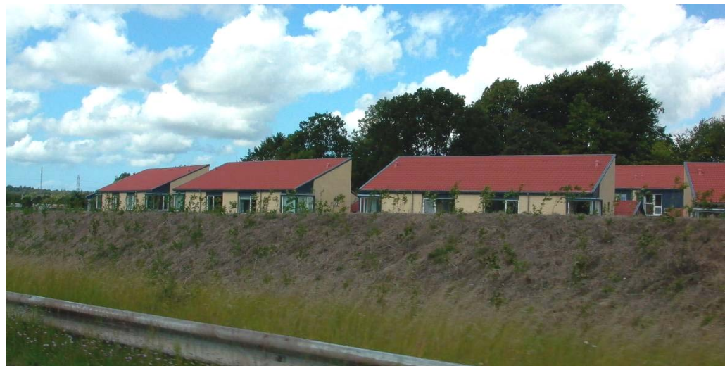
Figure 7.1. Earth embankment constructed at the same time as a new housing district to reduce the noise from an existing road at the houses and the gardens at Kvistgård, Denmark.
