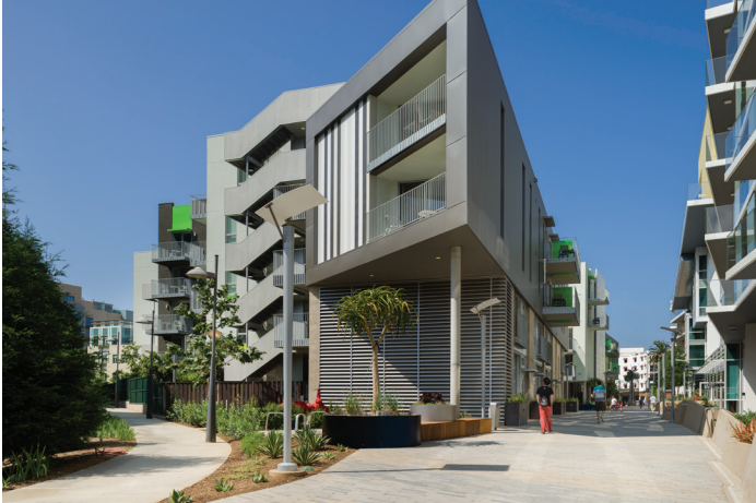
Western Courtyard with Pavilion
