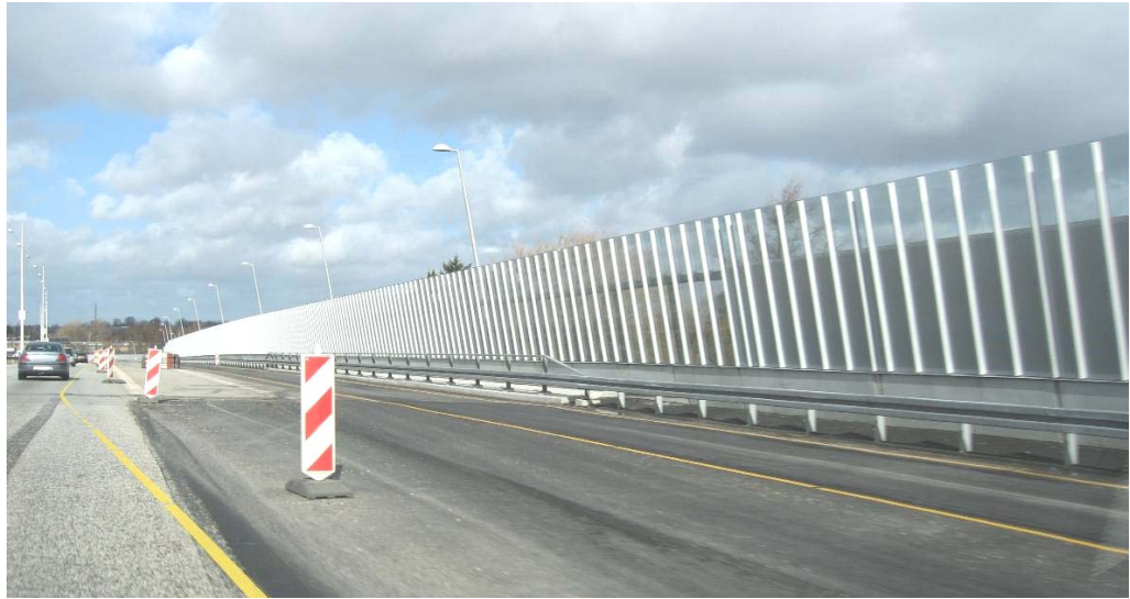
Figure 5.2. 3 to 4 m high noise barriers have been constructed along highway M3 as part of the enlargement project.
