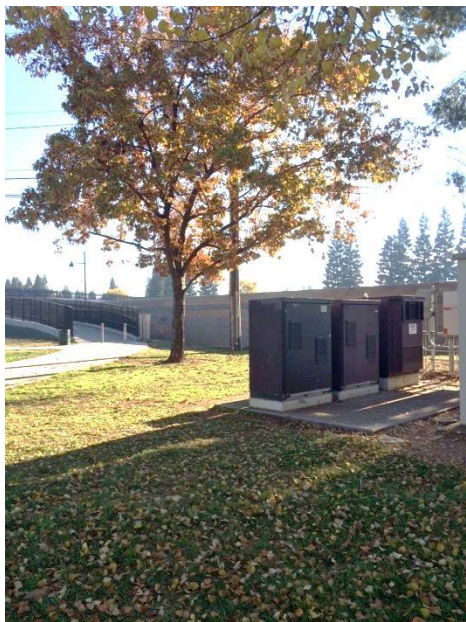
Frequent Encampment Area in White Rock Park next to the Pedestrian Bridge
