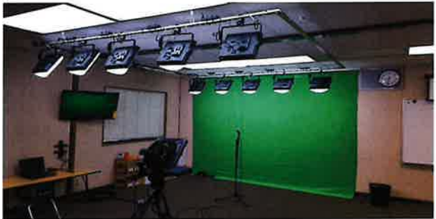
Example of light mounting solution using Unistrut/superstrut suspended a few inches below false or T-bar ceiling
