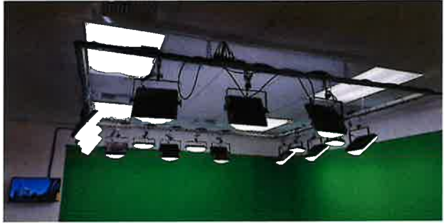
Example of light mounting solution using Unistrut/superstrut suspended a few inches below false or T-bar ceiling
