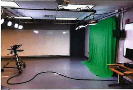
Single camera / teleprompter / monitor set-up with green screen shooting area. Lighting is staged rear to front for 1) green screen background, 2) hair light, 3) talent light
